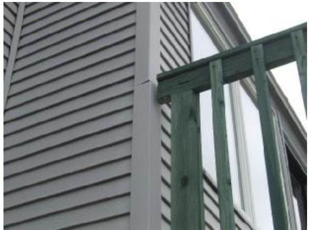
This corner trim should overlap to keep water out.
