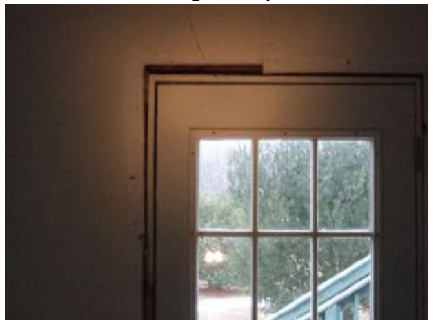
Trimming this door will help keep a draft out.
