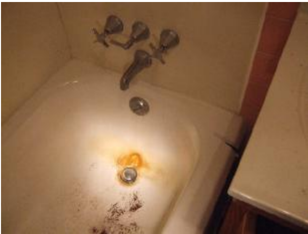
The staining of the tub could mean water with a high mineral content.
