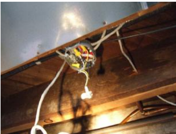
Exposed wiring.
