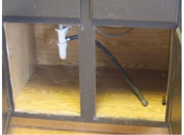
This line may have been a discharge for a dishwasher.
