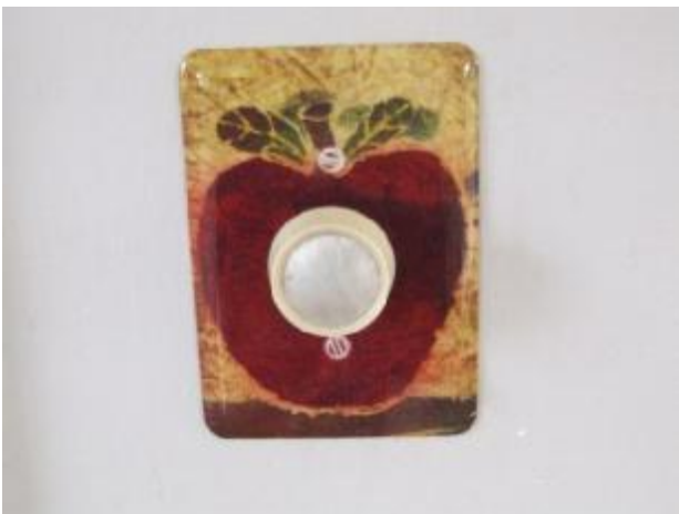
The light operated by this dimmer is fluorescent. This won't work. It needs a flood light.
